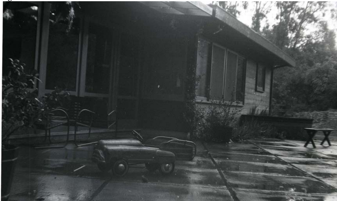
Photograph of play car on patio, March 1958, latticed eaves, boxed eaves, gallery window wall, dining room windows, redwood siding, kitchen window, and concrete patio with redwood latticed inlay visible. Photograph courtesy of Theodore Thomas, Jr.
